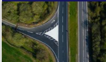
Road & Rail restoration works from Daniel storm
